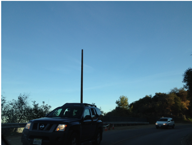
New cell pole on Mulholland Drive
